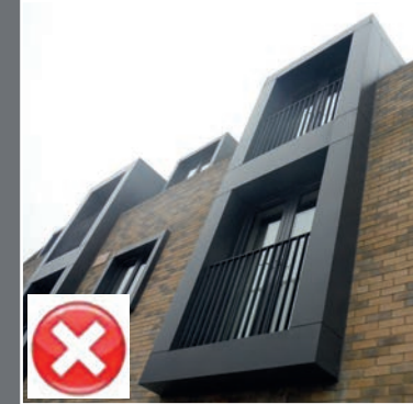
All too often balcony spaces are provided but are rendered unusable due to their small size, orientation to the north or proximity to highly trafficked and noisy roads.
