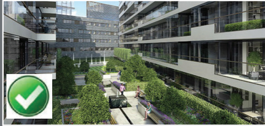
A high density scheme with generous communal space and balcony provision
