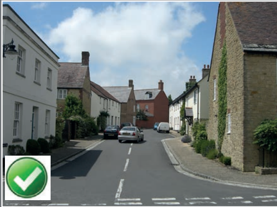
Street with an interesting & rich roofscape
