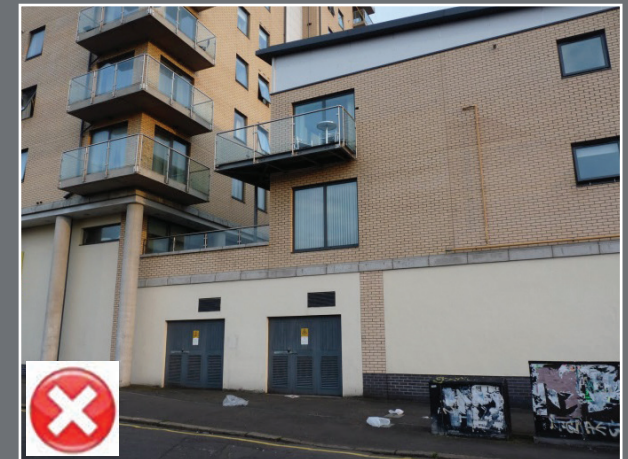
An inactive frontage with a largely blind façade at street level
