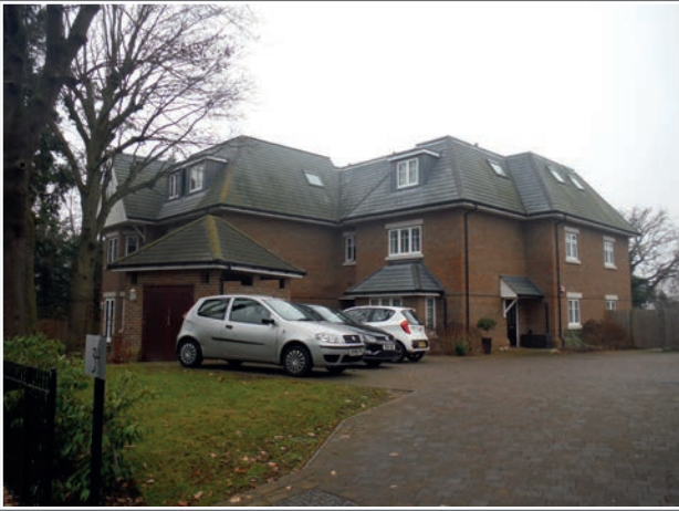
An overly deep building with an awkward roof form
