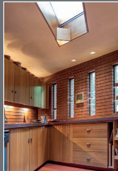
Domestic kitchen lit by slit windows and rooflights
