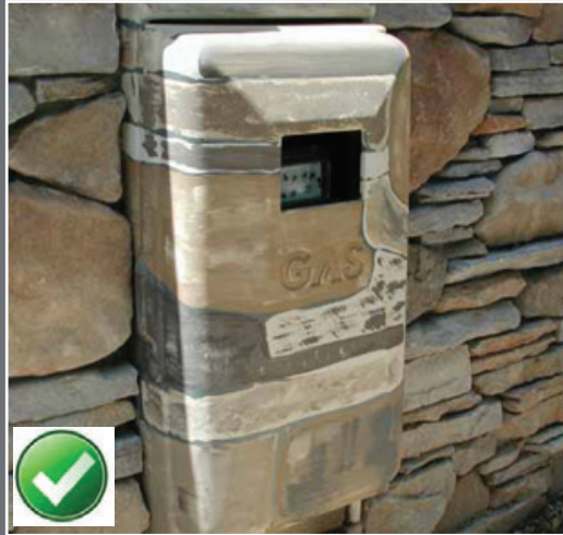
Cabinet design that blends with the house materials
