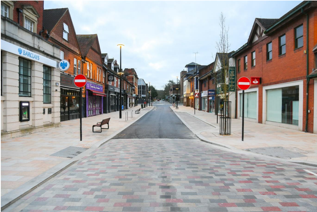
Camberley Town Centre Improvements
