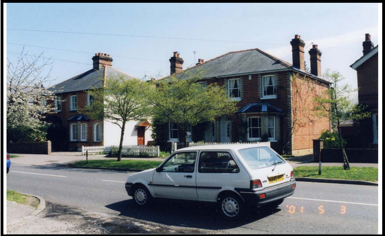
9. Castle Grove Road villas.
