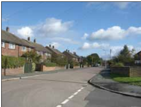
Flat elevations, regular building lines and brick walls
