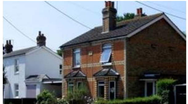
Benner Lane Early 1900s cottages with sash windows.
