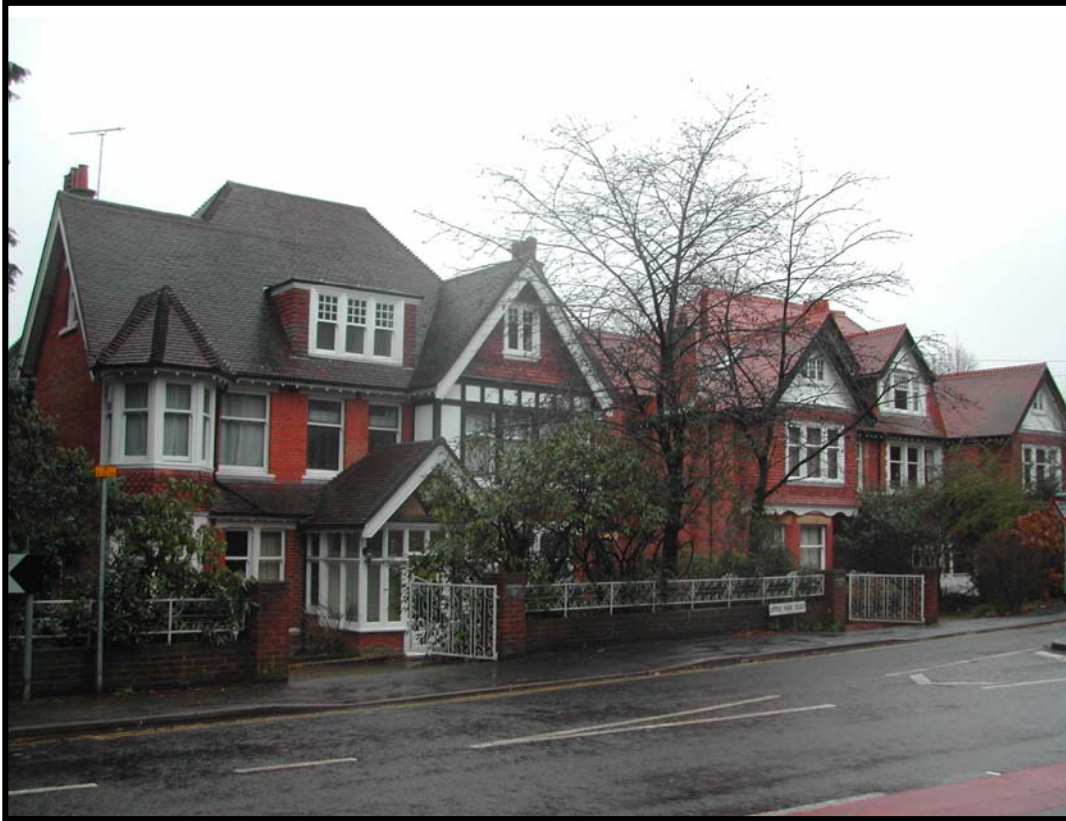
5. 37, 39, 41 Upper Park Road (west). Jan. 04
