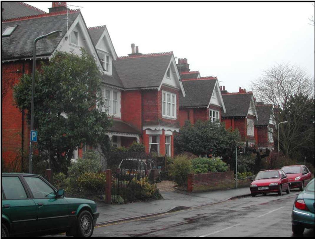
3. View of properties to south side of Upper Gordon Road. Jan. 04
