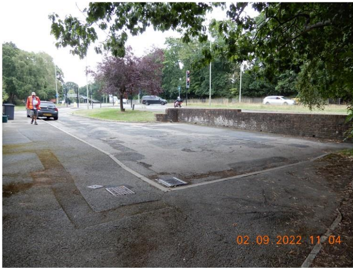
Photograph 1 — Eastern site boundary where it abuts Caesar's Close.
