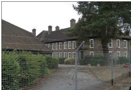
Image 6.7 North east view of the Director of Logistics HQ building
