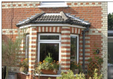
Decorative brickwork - West End
