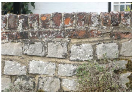
Brick and stone walls
