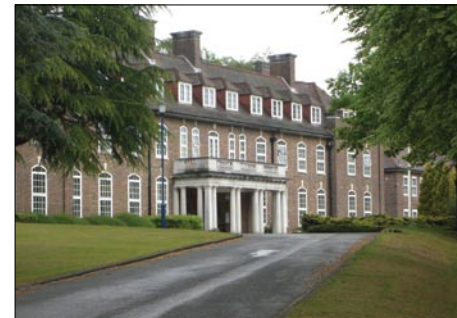
Former officer's Mess, Deepcut
