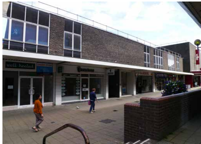
Large footprints in the core of the town centre can be inflexible to changing demands and uses
