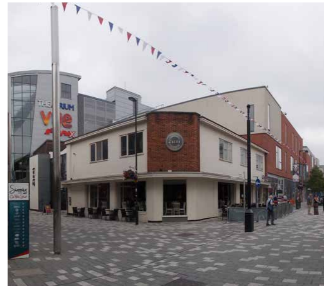
Existing condition - Park Street.
