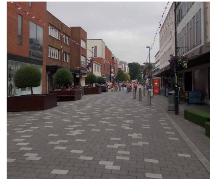
Existing condition - Park Street.
